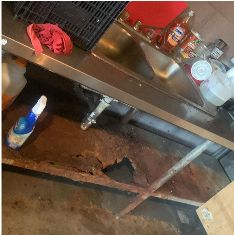
Figure 18. Farmworker Kitchen Conditions
